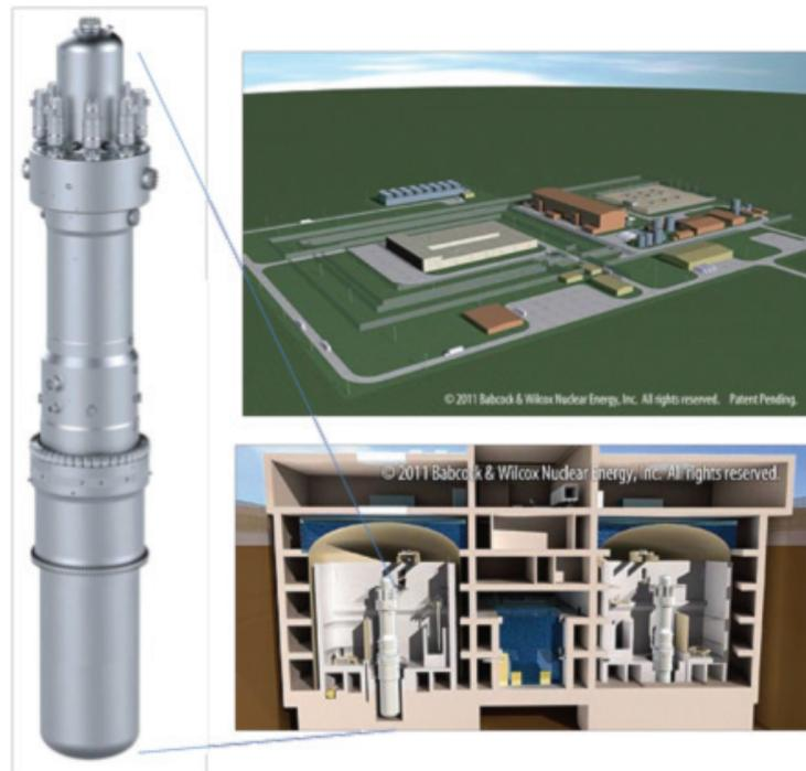
FIGURE 3 Illustrates the Reference Westinghouse 225 MWe SMR Plant with one module, Details of the Below Grade Containment and Integral Pressure Vessel
