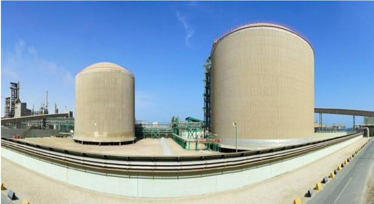
*Two 50,000 metric tons net capacity single-wall refrigerated ammonia storage tanks built by McDermott in Messaieed, Qatar<sup>41</sup>; these tanks hold ammonia with an energy content of around 2 million MBtu. (Picture: HansonDoha)*
