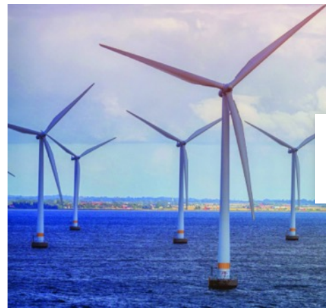
2.5 GW offshore wind (Largest offshore wind facilities today ~ 1 GW)
