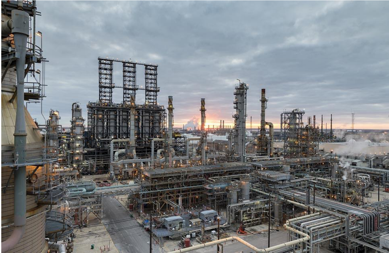
Valero Oil Refinery in Port Arthur
