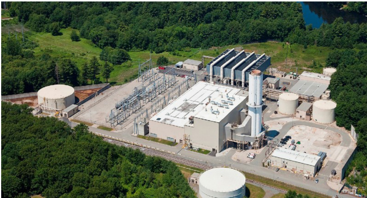
Bellingham Power Plant Source: NextEra Energy
