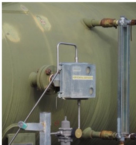
A shows the liquid level controller with a regular camera, where emissions are invisible; B shows the same liquid level controller captured using an OGI camera, where emissions are visible in green. The equipment should be venting less during normal operations.
